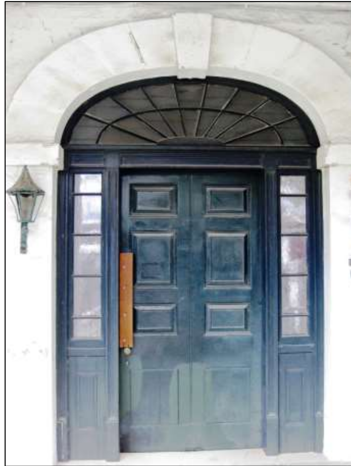
Figure 2 Cleveland House front door
