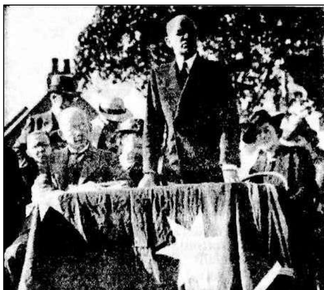
Figure 13 Opening of Shannon Reserve ( Sydney Morning Herald , 21 August 1939)
