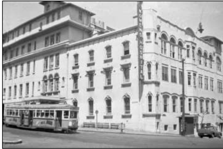
Figure 28 Crown Street Women's Hospital, 1958 (City of Sydney Archives)
