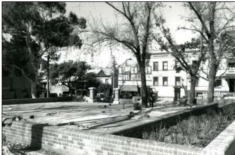
Figure 20 Shannon Reserve construction, 1990s (City of Sydney Archives)
