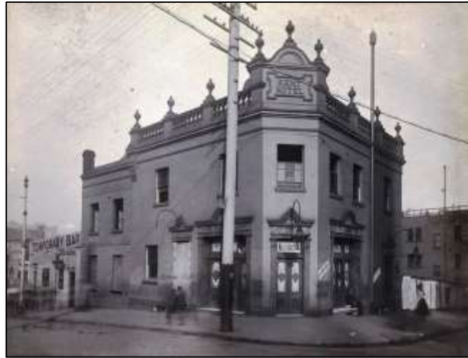
Figure 61 Kent Hotel, 1907 (City of Sydney Demolition Books)
