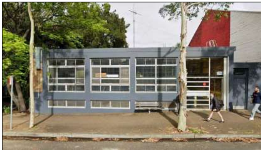
Figure 66 549 Dowling Street, 2022 (Google maps)
