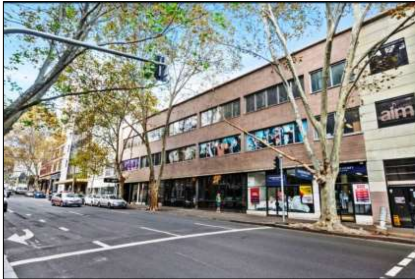
Figure 51 Former Senatorial Hotel site today ( realcommercial.com.au )
