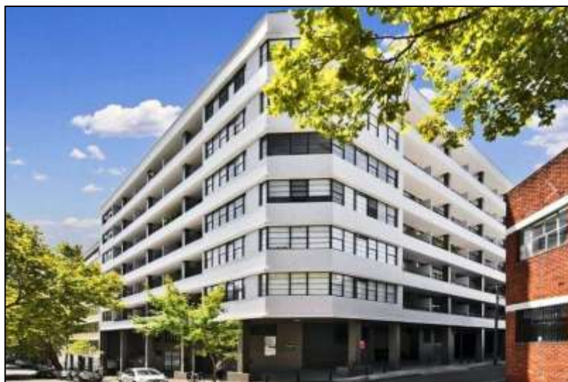
Figure 53 Former Standard Hotel site today (traversgay.com.au website)
