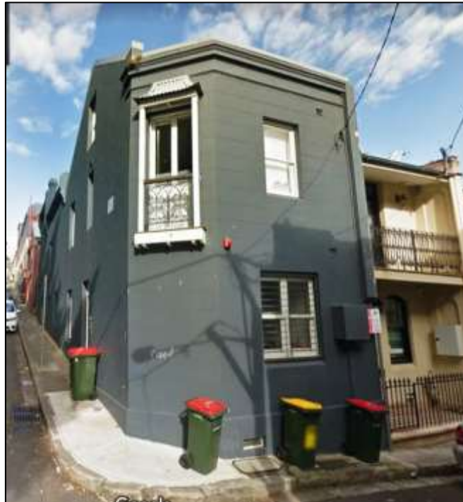
Figure 28 Former Lloyd's Hotel today
