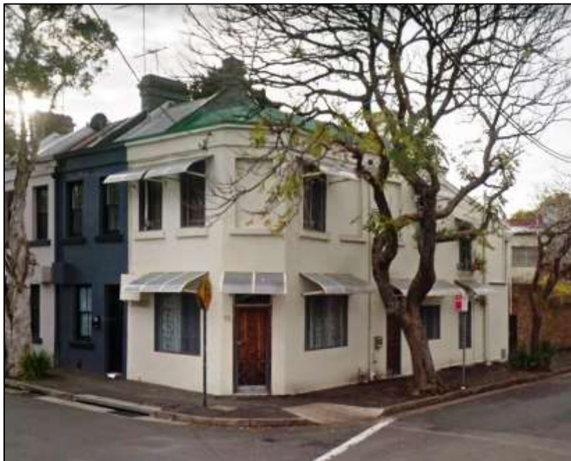
Figure 36 76 Marshall Street, 2015 (Google maps)
