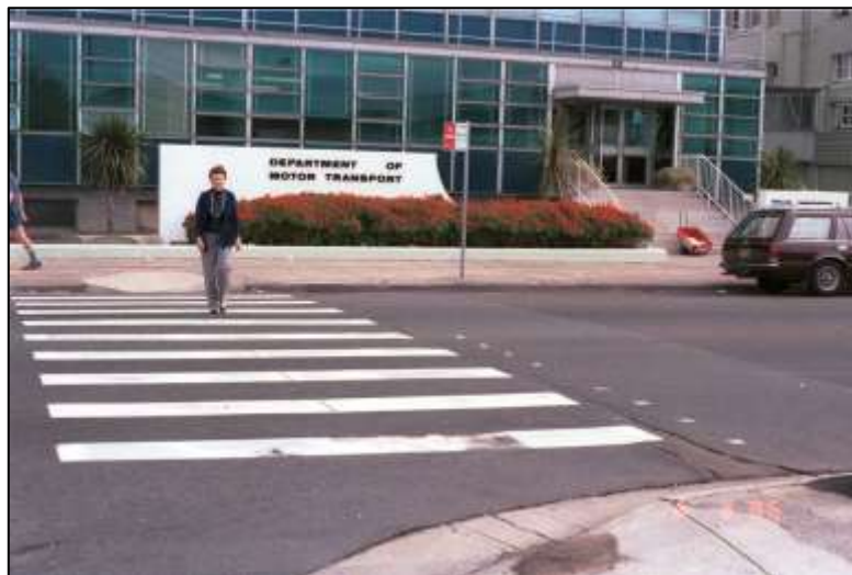
Figure 19 DMT Motor Registry building, 1986 (City of Sydney Archives)
