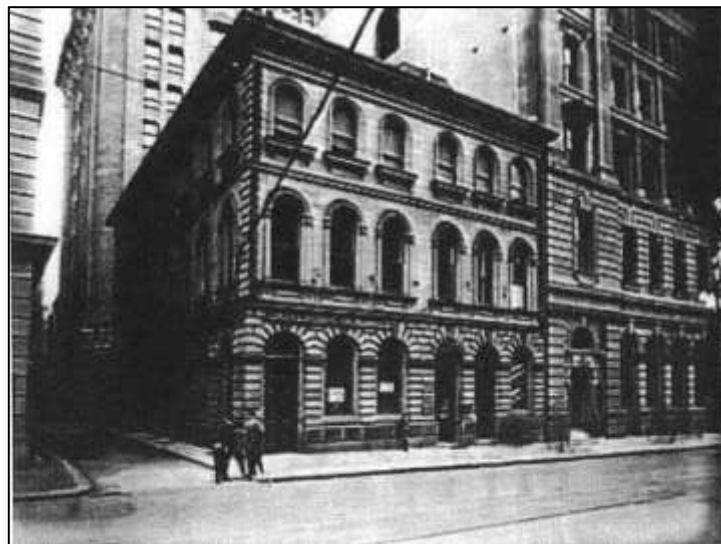
Figure 25 Original 1860 building, Pitt St, 1916 (City of Sydney Archives)
