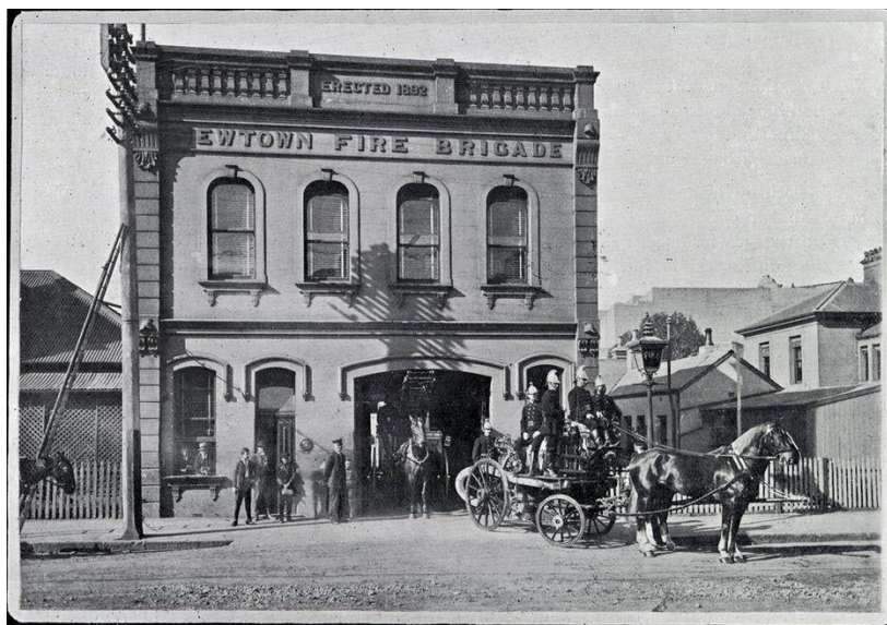
Figure 25 Newtown Fire Station, 1912 (City of Sydney Archives)
