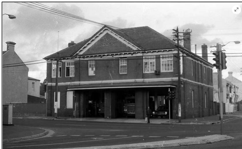
Figure 28 Waterloo fire station, 1973 (Museum of Fire)
