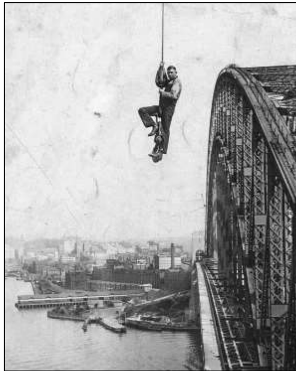
Figure 56 Building the Harbour Bridge (Bridge Climb website)
