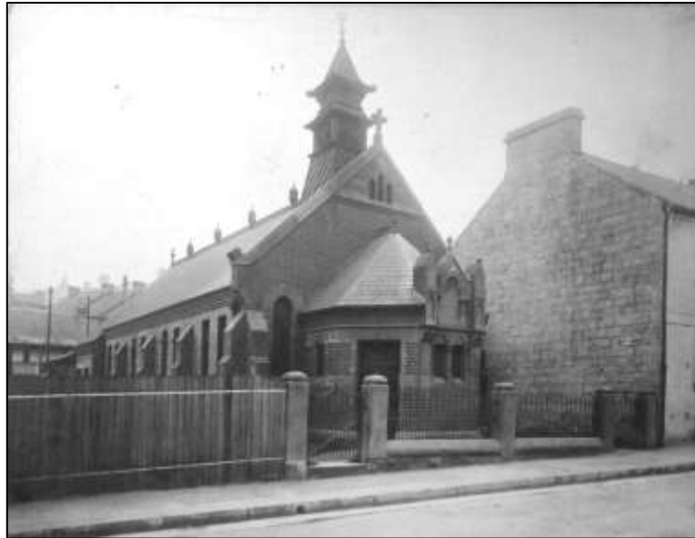
Figure 24 St Luke's Anglican Church, c1908 (City of Sydney Archives)
