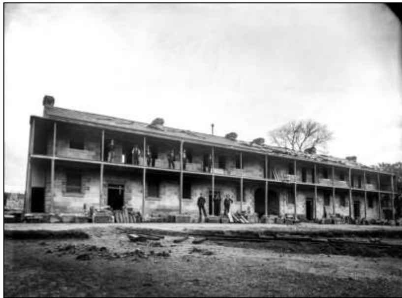
Figure 18 Demolition of the Police Barracks, 1901 (City of Sydney Archives)
